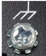
*Figure 2.15 - Grounding screw*
